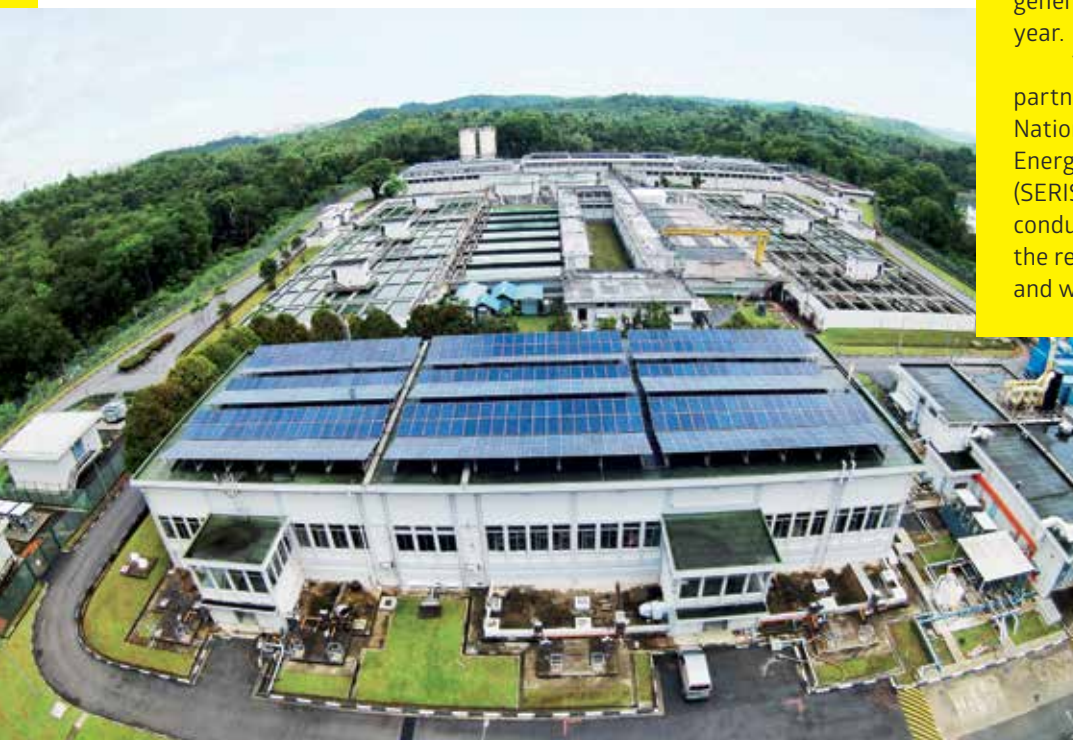
Left: Solar panels at the Choa Chu Kang Waterworks
