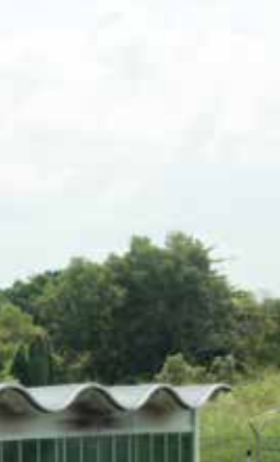
Left: NEWater storage tank
