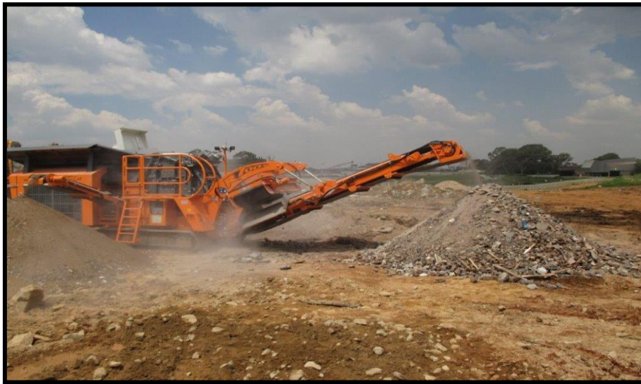
Figure 5-2: Builders' rubble crushing at Robinson Deep landfill
